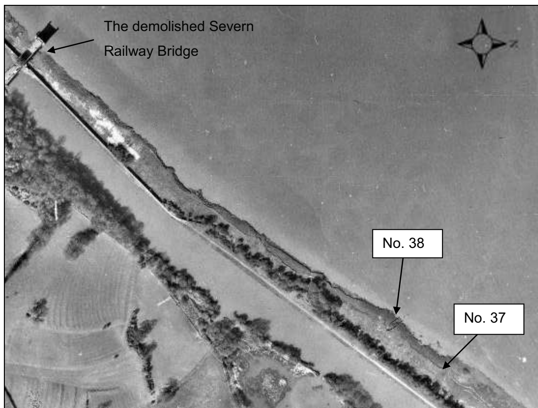
Figure 7. The breakwaters in 1969.
